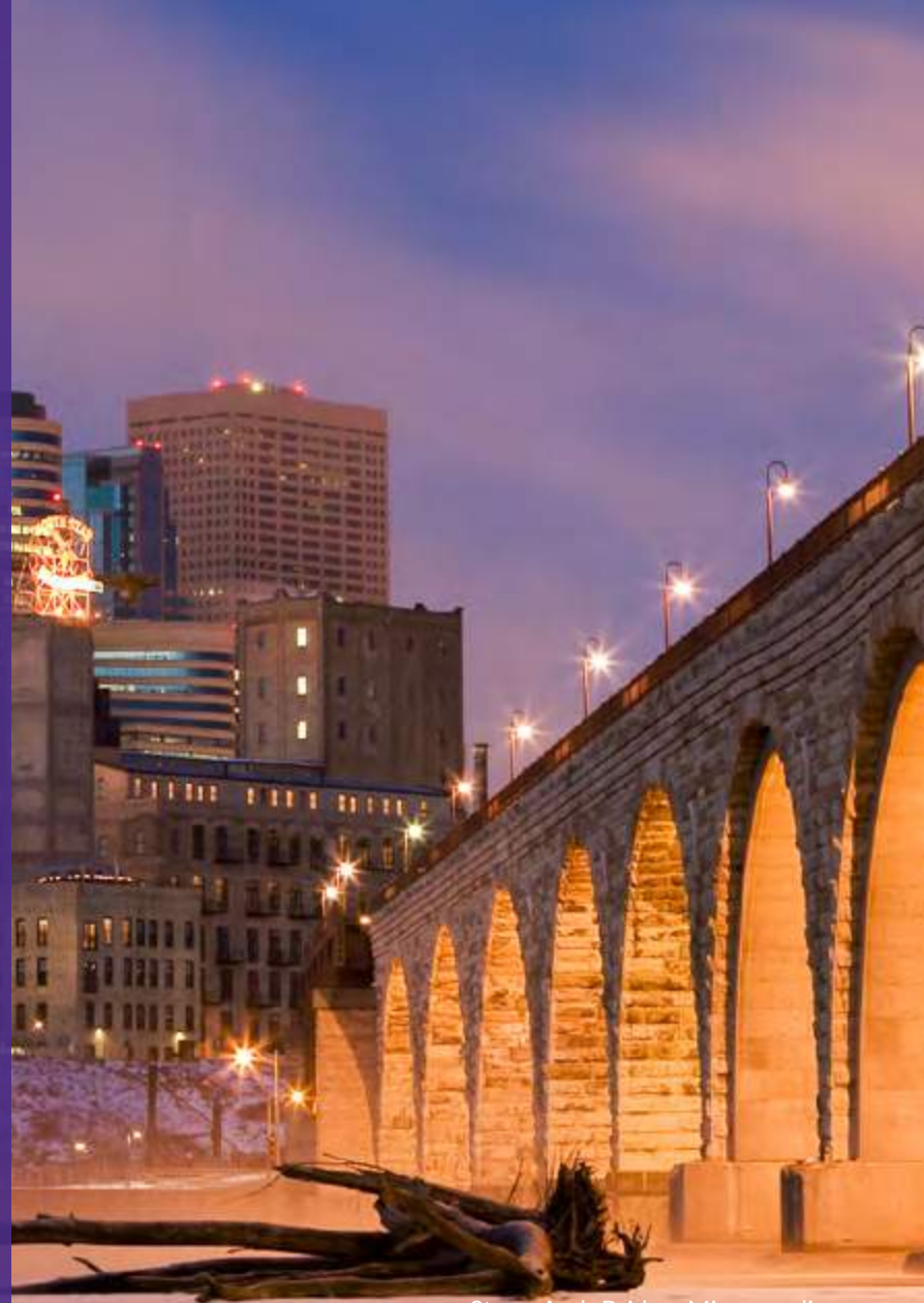
Stone Arch Bridge, Minneapolis
